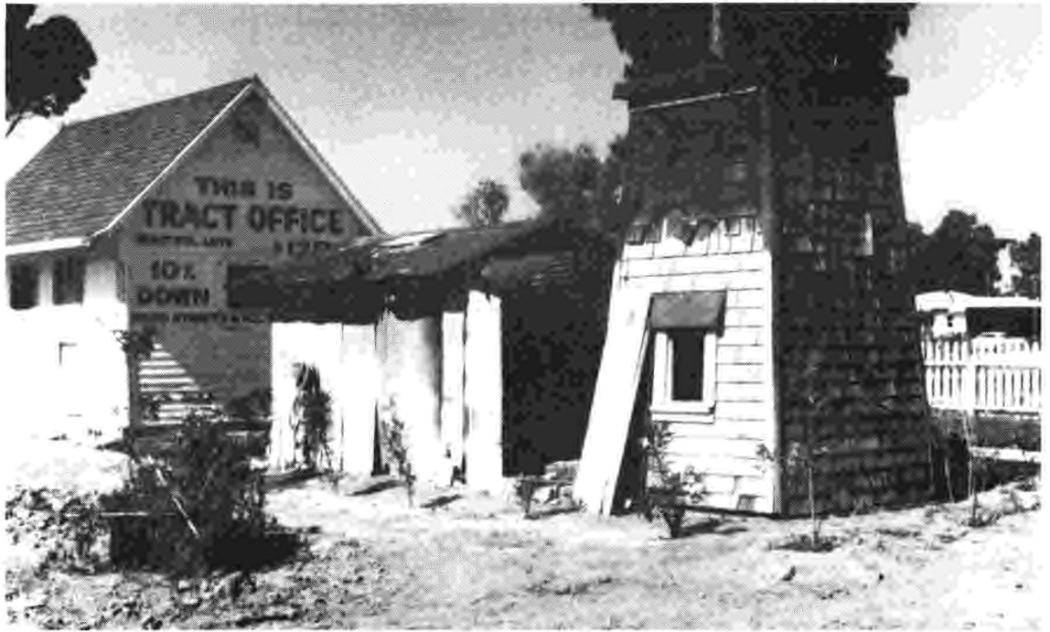
The old Talbert Real Estate Office shown with the Japanese bath house and water tower
