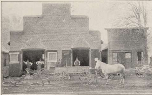
OFFICE AND BLACKSMITH SHOP OF J. T. WYLIE. Photo by Matthews.
