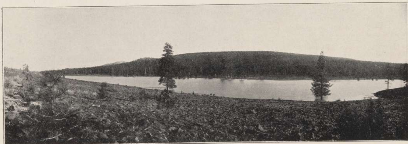
RESERVOIR BUILT BY IMIRIE & TORRESON.
