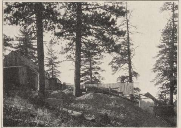
SHAFT HOUSE, HESS MINE.
