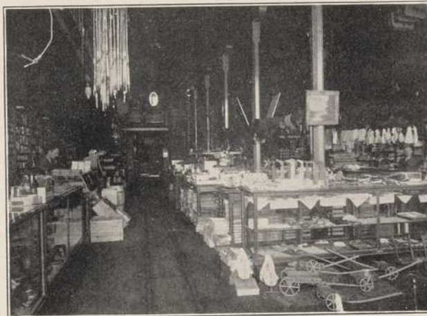
INTERIOR OF GEO. H. KNIGHT'S EMPORIUM AT ADIN.
