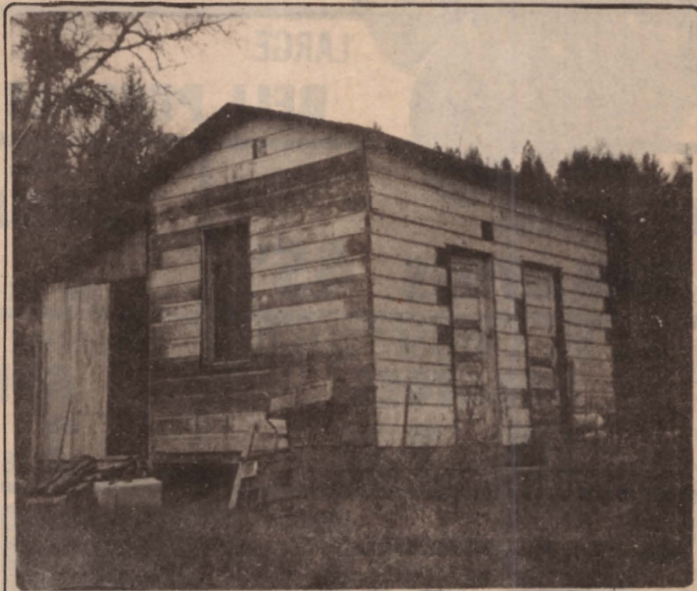
The Farley School is shown as it looks today. It is on the west side of Highway 101 a couple of miles south of Laytonville.
