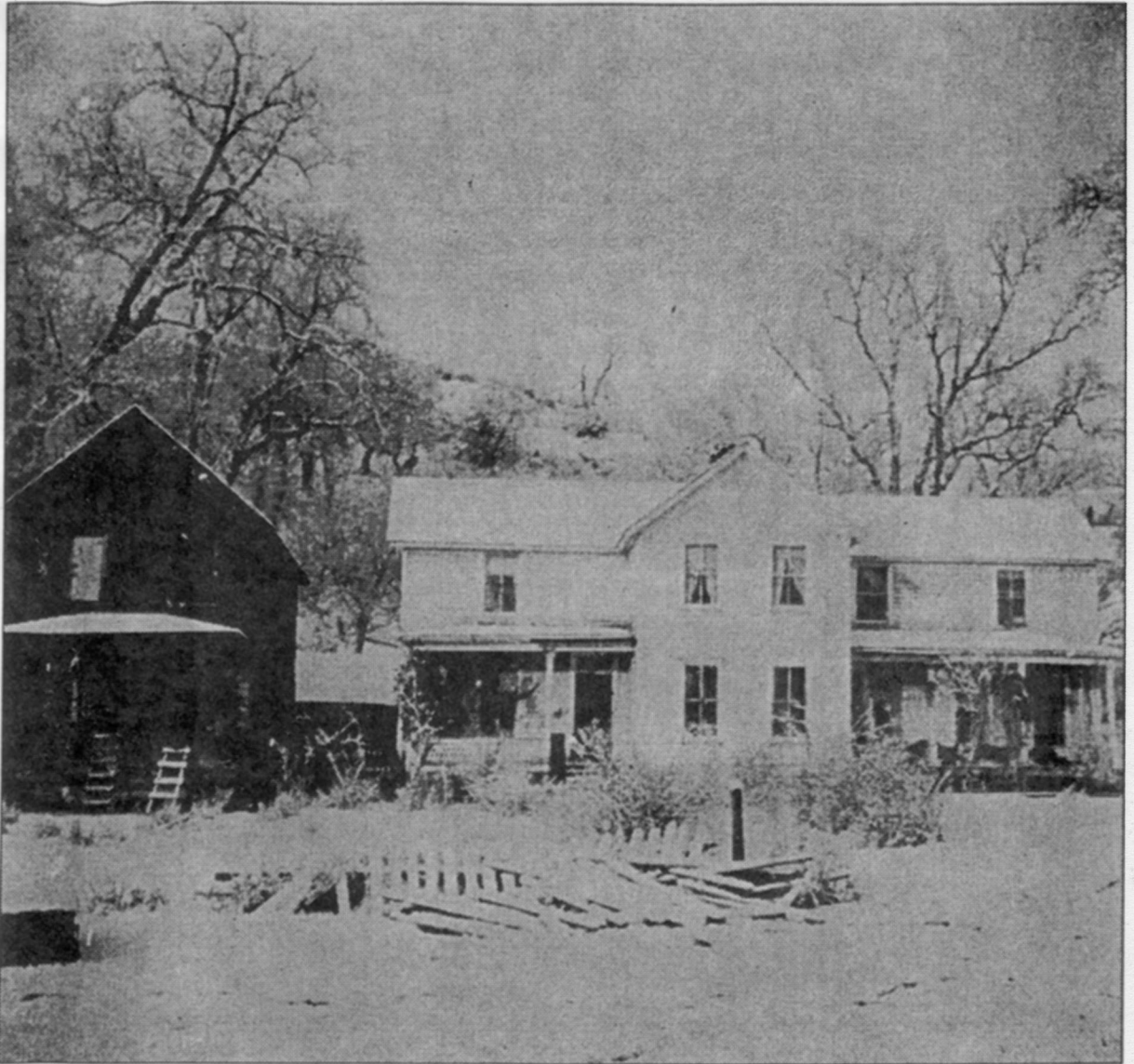
Eden Valley Ranch main house where the ranch hands ate their meals. Next to the house is one of the original buildings on the ranch probably built around 1870.
